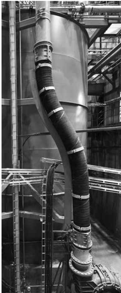
Picture 2: Material handling hose with support beam and clamps
